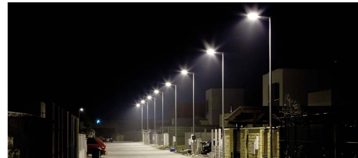
In the top image, the light sources emit perceptibly different light colours. Although this phenomenon does not noticeably affect visual acuity, it is aesthetically displeasing.
