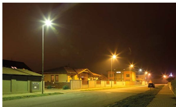
These two photographs show similar streets. On the left is a street illuminated by an old lighting installation, and on the right, another street after the lighting was renovated using modern luminaires and white light sources.
