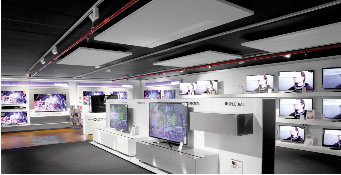
The combination of continuous line linear lighting fixtures and accent lighting spotlights means that both general and accent lighting are simply and effectively provided in a low maintenance, flexible and practical way.
