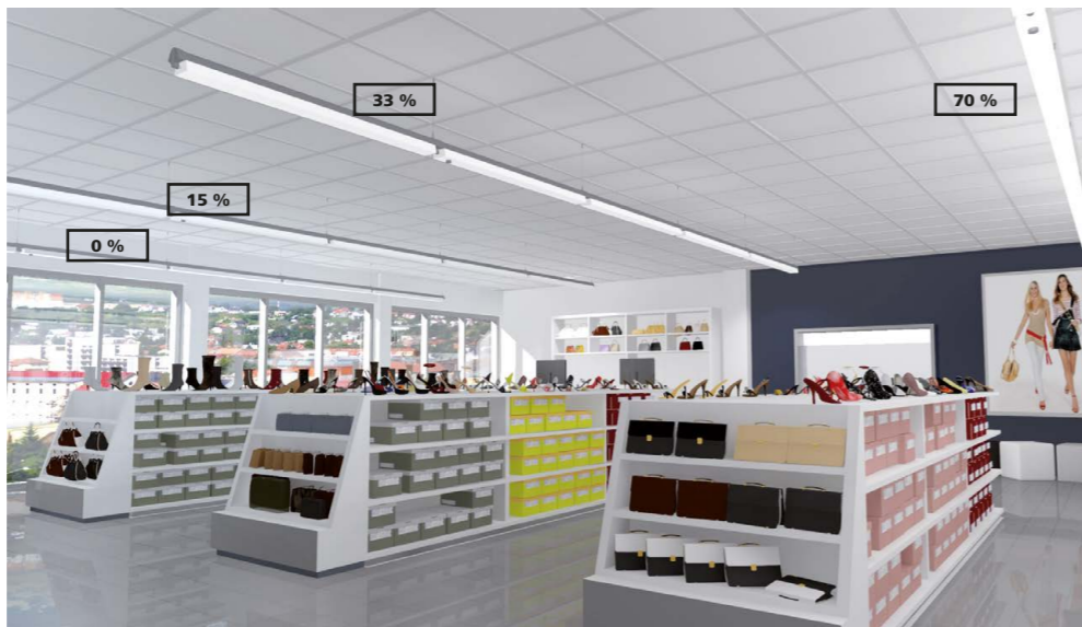
If the room has large windows and during the day there is sufficient daylight it is suitable to use cascade scanning to dim the luminaires. For maintaining a uniformity of lighting throughout the whole space the luminaires are automatically dimmed more at the windows.
