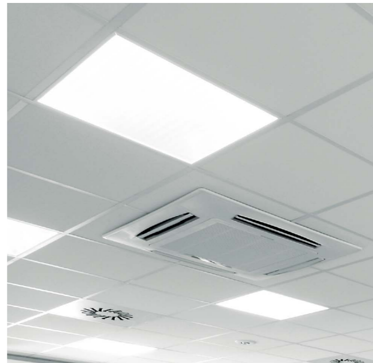
It is approximately valid that for 2.5 W of the luminaire energy 1 W of the air-conditioning energy is used, i.e. if the energy consumption of the lighting system increases, the energy consumption for the air-conditioning operation grows in direct proportion, too.
