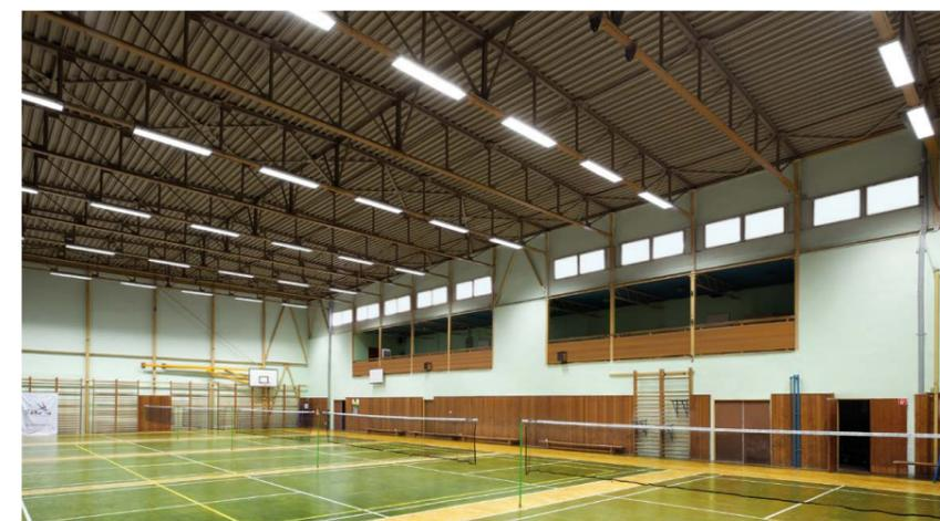
When planning the illumination of the sports facilities, intensity and uniformity of the lighting are the most important criteria.
