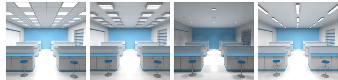
When selecting the luminaires for the labs and workshops it is necessary to take into account several factors at the same time. It is suitable to use luminaires with the protection level IP 54 or IP 65 in these spaces. In the workshops where there is a higher risk of injuring by moving rotating or reciprocating machines the luminaires should be fitted by electronic control gears to prevent the rise of the stroboscopic effect.
