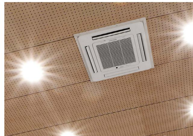
It is approximately valid that for 2.5 W of the luminaire energy 1 W of the air-conditioning energy is used, i.e. if the energy consumption of the lighting system increases, the energy consumption for the air-conditioning operation grows in direct proportion, too.
