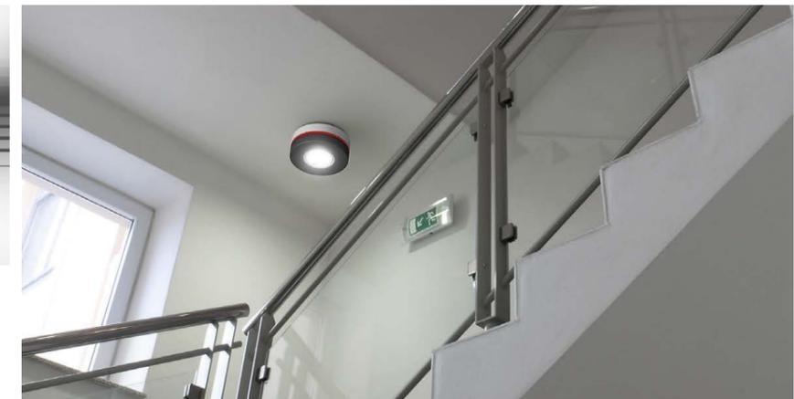
During normal operation the illumination level of communications zones reaches prescribed levels. During the blackout or in case of fire emergency lighting ensures the pupils basic visibility and orientation during leaving the space or to make their access to the fire extinguishers easier.
