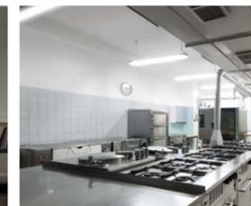
*For lighting the kitchens of the mass catering establishments the standard EN 12464-1 determines the minimal illuminance level 500 lux. The luminaires have to possess sufficiently high colour rendering index CRI, to be resistant against high temperatures, vapour and chemicals. It is recommended to use unbreakable luminaires over the area for preparing meals or luminaires protected by a special cover which will prevent the fragments from falling onto the meals if the luminaire is damaged.*
