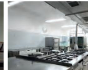
For lighting the kitchens of the mass catering establishments the standard EN 12464-1 determines the minimal illuminance level 500 lux. The luminaires have to possess sufficiently high colour rendering index CRI, to be resistant against high temperatures, vapour and chemicals. It is recommended to use unbreakable luminaires over the area for preparing meals or luminaires protected by a special cover which will prevent the fragments from falling onto the meals if the luminaire is damaged.
