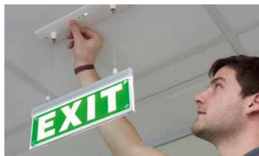
Smaller installations that have no central monitoring system need to be regularly tested manually.
