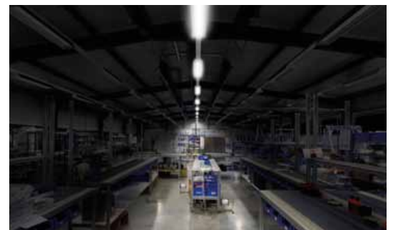
Outside of working hours the lighting can be dimmed to a safety level suitable for monitoring.
