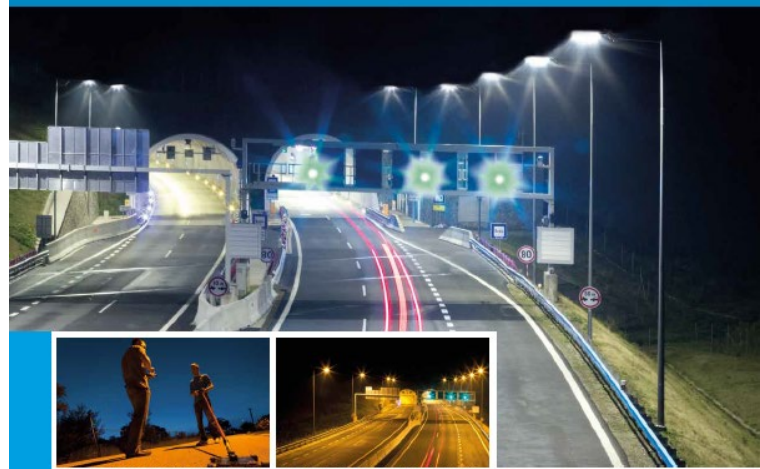
Even the smallest reconstruction does not mean no major requirements.
