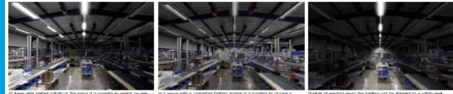
All areas with linked activity in the space it is possible to switch on only the equipment needed in the necessary location by selecting the outdoor lighting zones according to production and energy activity of for a time. In a space with a control lighting system it is possible to choose a lighting scene according to production and energy activity of for a time. Outside of working hours the lighting can be directed to a safety area without any monitoring.
